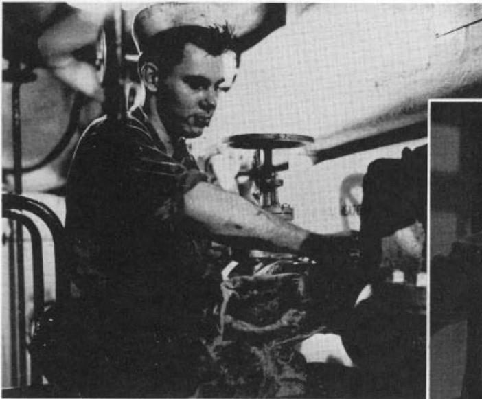
Cutting in the fuel oil heater
